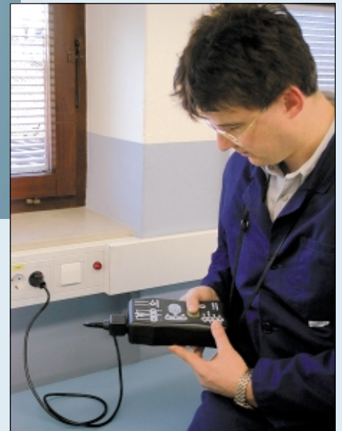
All the tests are done directly at the socket
